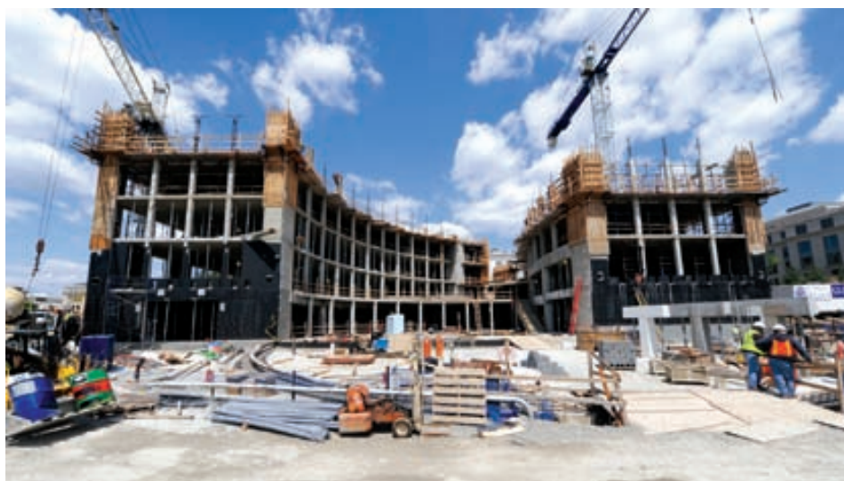
United States Institute of Peace Headquarters under construction, April 2009.
